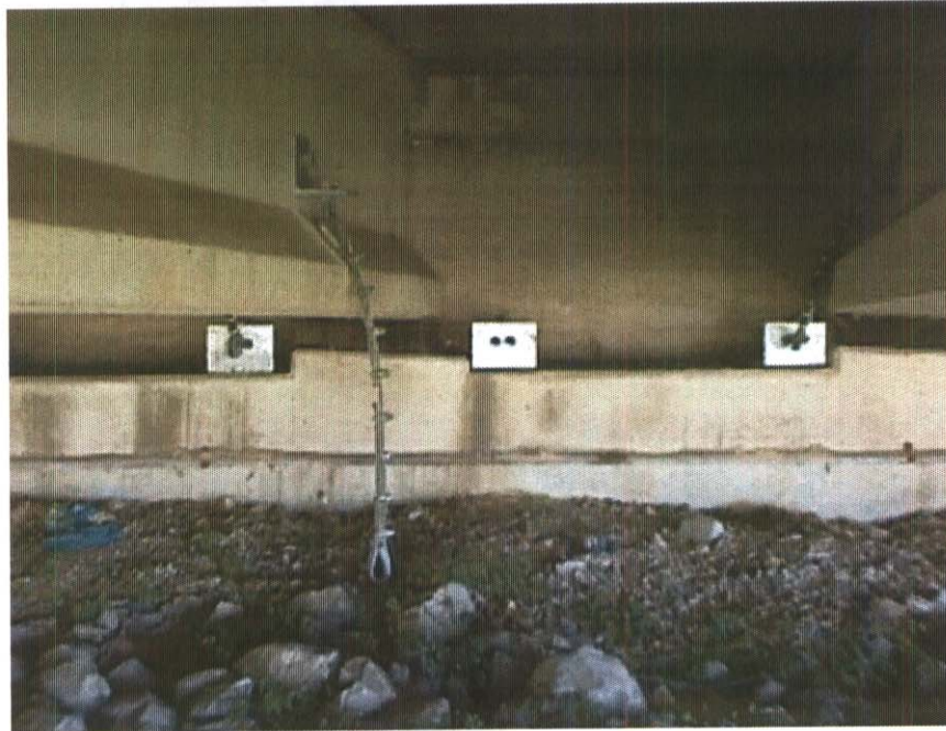
ABUTMENT #1 EARTHQUAKE CABLE CONNECTED TO GIRDER "D", BROKE LOOSE
