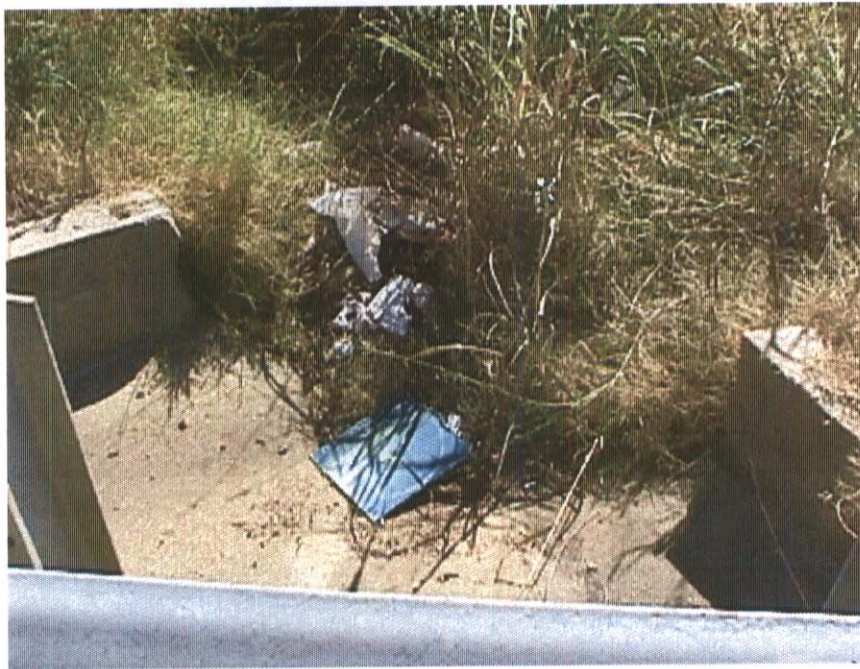
APPROACH #1, BROKEN DRAIN CURBS
