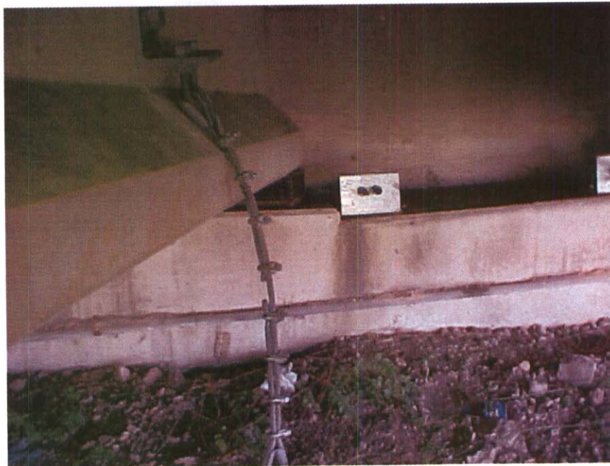
SPAN #1 EARTHQUAKE DEVICE IS BROKEN
