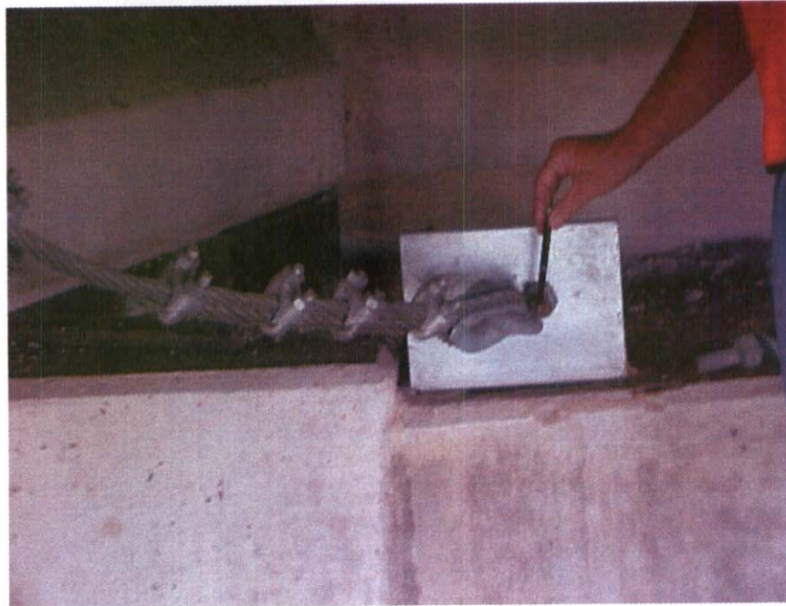
SPAN #1 EARTHQUAKE DEVICE IS BROKEN
