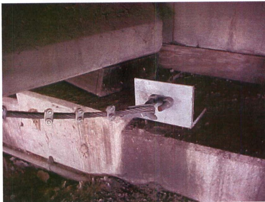
SPAN #1 EARTHQUAKE DEVICE IS BROKEN
