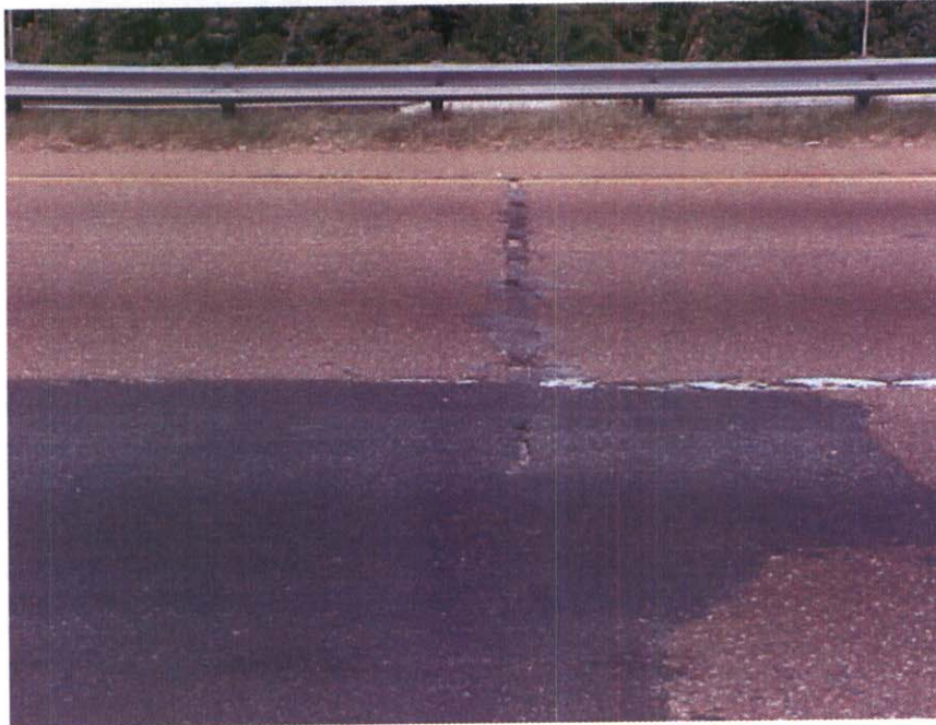
APPROACH #1 HAS JOINT MATERIAL MISSING, TYPICAL OF APPROACH #2
