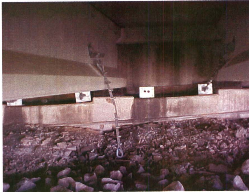
SPAN #1 EARTHQUAKE DEVICE IS BROKEN
