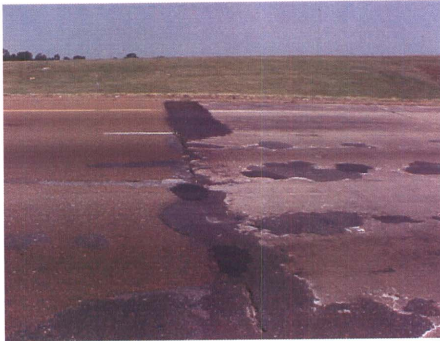
APPROACH #2 ASPHALT SPALLING
