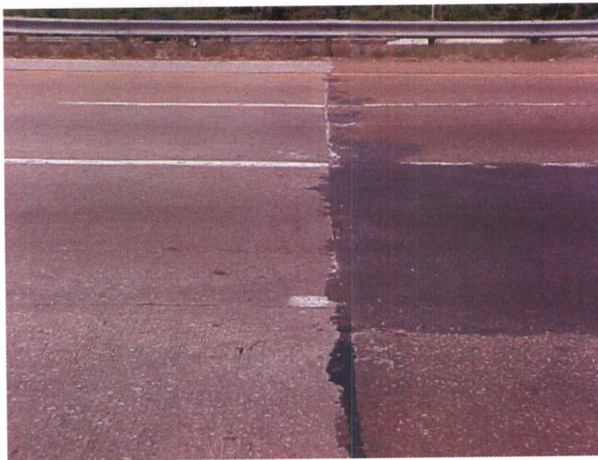
APPROACH #1 HAS JOINT MATERIAL MISSING, TYPICAL OF APPROACH #2
