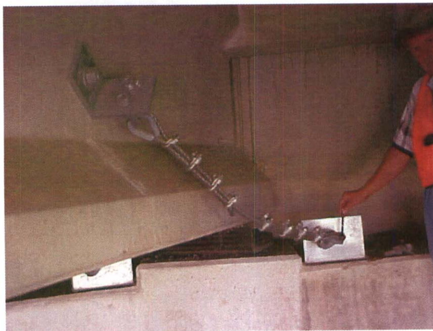
SPAN #1 EARTHQUAKE DEVICE IS BROKEN
